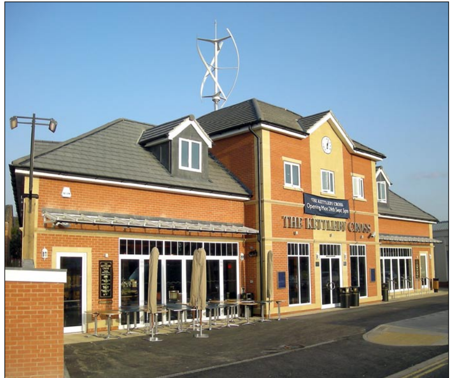
Good head on the glass: Wetherspoon expects payback from the installation of the first ever roof-mounted quietrevolution wind turbine
